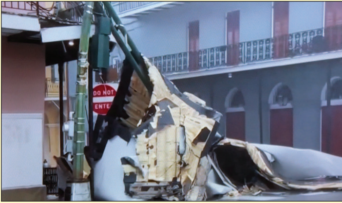
In this TV image, a roof has collapsed in New Orleans
