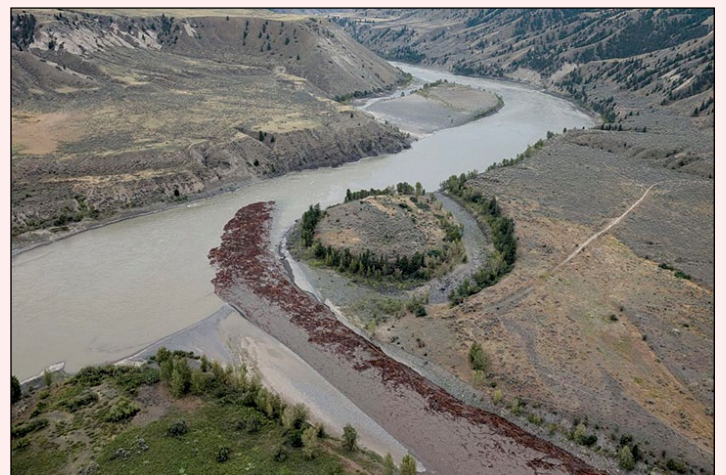
Figure 4 - The leading edge of the floodwater after it broke through the dam on August 5. Photo provided by EMCR
