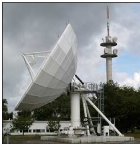
MSG Receiving Antenna and Microwave Tower
