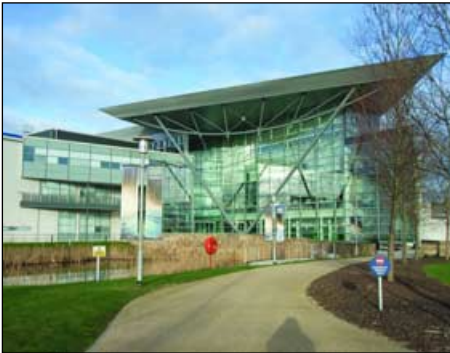
Figure 6 - Met Office HQ in Exeter
