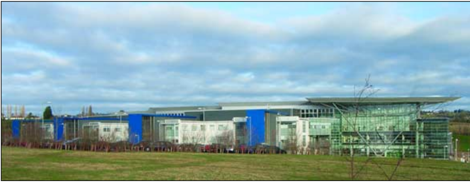
Figure 4 - Met Office HQ in Exeter
