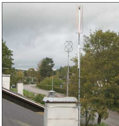
Figure 6 - Twin antennas for 'diversity' reception
