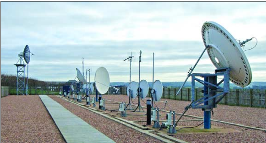
Figure 9 - The Met Office Antenna Farm
