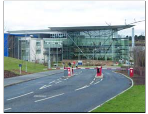
Figure 5 - Met Office HQ in Exeter
