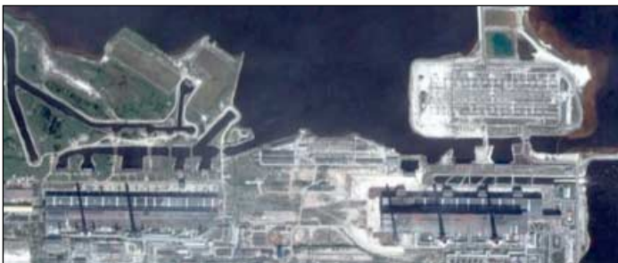
Figure 7 - The Surgut power stations, with their giant flues evident.
