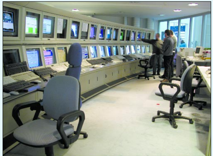
The Meteosat Transitional Program (MTP) control room
