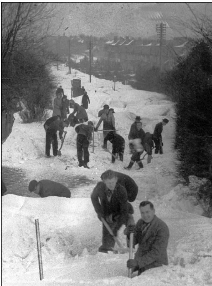
Figure 6 - Digging through snow drifts to keep the A456 Kidderminster to Birmingham road open.
