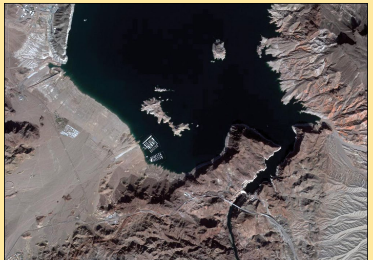
The south end of Lake Mead with the Hoover Dam Modified Copernicus data © ESA / Sentinel (2016)
