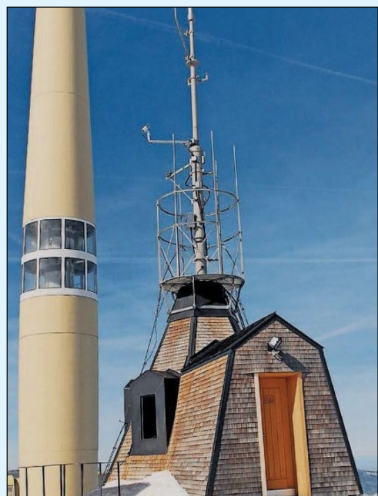
Figure 3 - The original meteorological station stands beside the present-day transmitting tower
