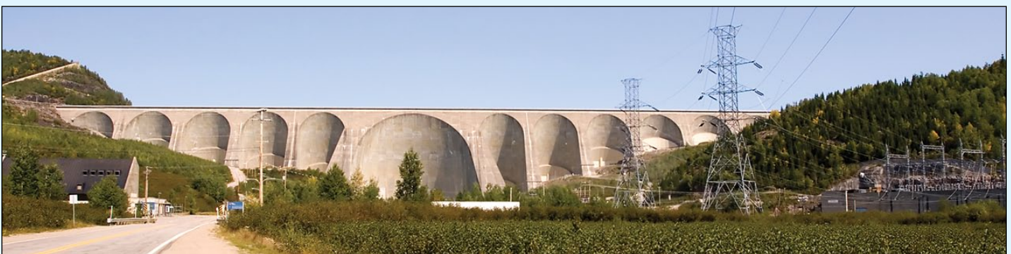
The 214 m tall, 1314 m long Daniel Johnson multiple-arch buttress hydro-electric dam on the Manicouagan River Image: Dan Fleet at English Wikipedia
