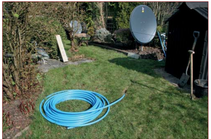
Figure 4 - Making use of MDPE piping for underground feeders
