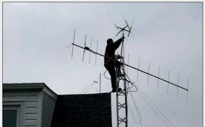
Steve up the mast installing the APT antenna
