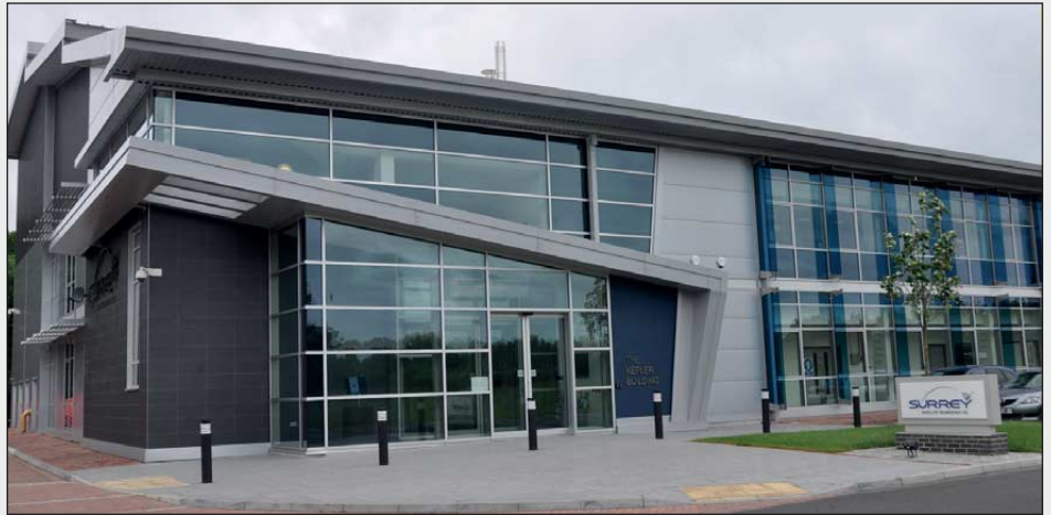
The SSSL satellite assembly building Photo: David Taylor
