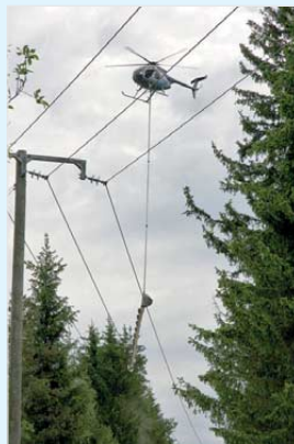
Figure 1 A Helicopter trims trees near a power line Image © Fortum
