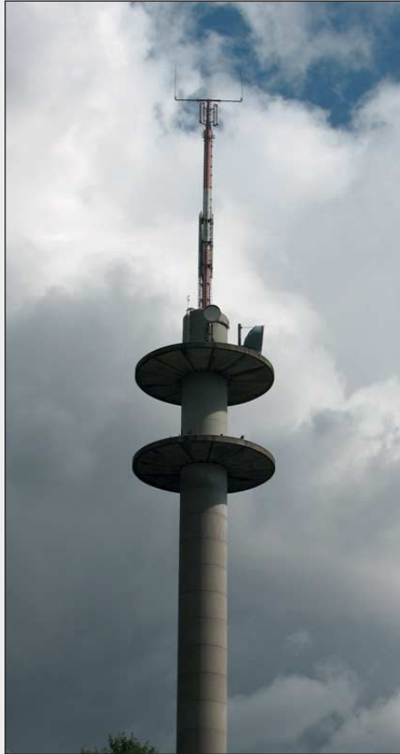
This radio tower provides microwave links between the ground station and MCC in Darmstadt
