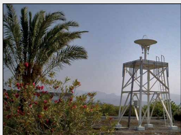
Figure 8 The Reception Antenna for EARS-AVHRR
