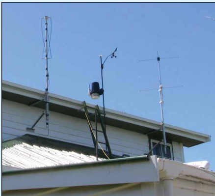
The author's roof with, QHA, Davis radio weather station (solar powered) and turnstile.
