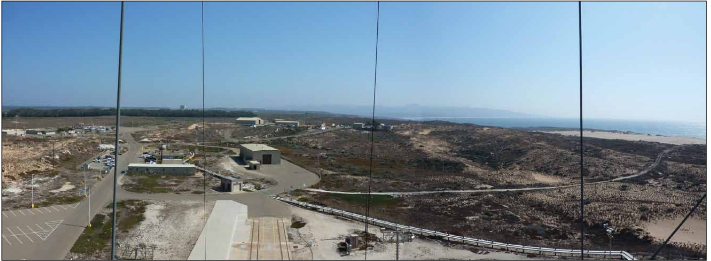
The view from Level 3. Ocean to the right, MST rails center bottom and Astrotech in the distance on the horizon.
