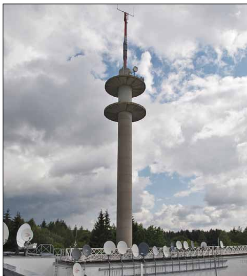
Figure 12 - The Usingen Transmission Tower
