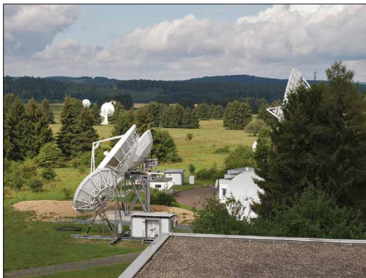
Figure 13 - An overview of the Usingen Antenna Park
