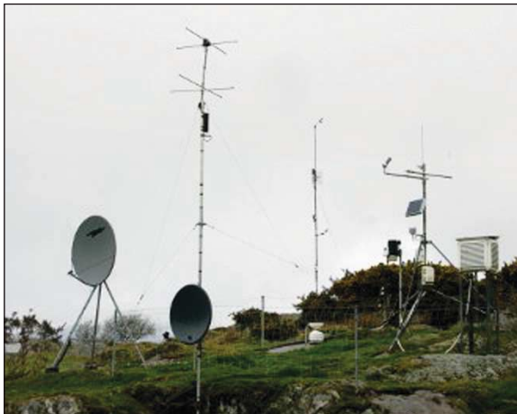
Fig 1 Automatic weather stations & antenna farm
