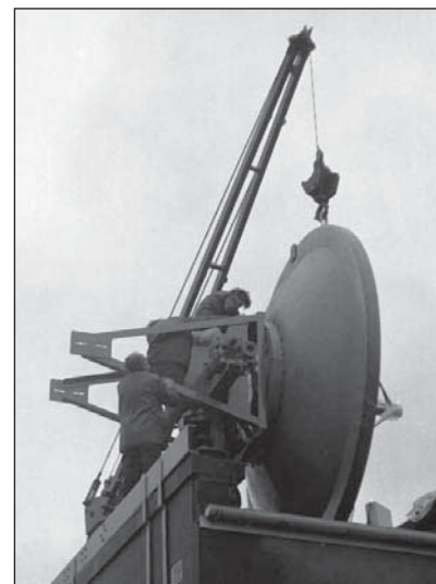
Figure 6 - Lifting HRPT antenna dish
