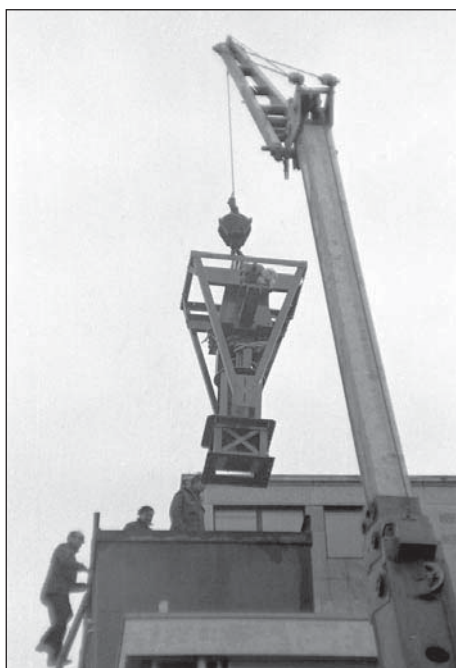
Figure 5 - Lifting the HRPT antenna base
