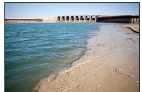
The spillway below the 13-kilometer dike at the southern edge of the Northern Aral Sea
