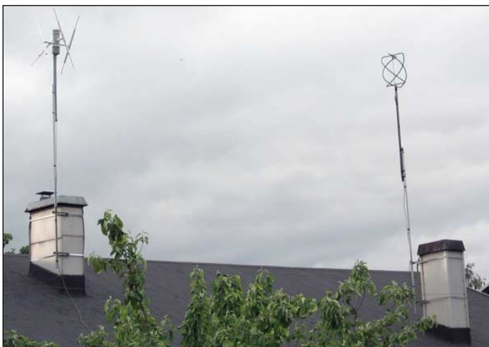
Figure 2 - Twin antennas for diversity reception
