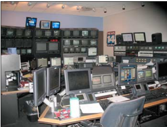
The control room at News 14 Carolina
